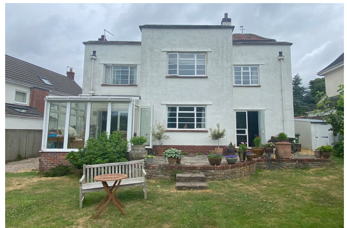
Views of rear elevation, existing conservatory, patio and steps down
