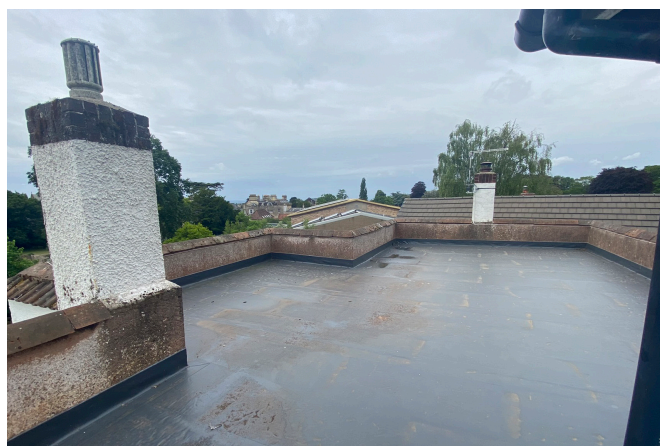
Existing flat roof and parapet
