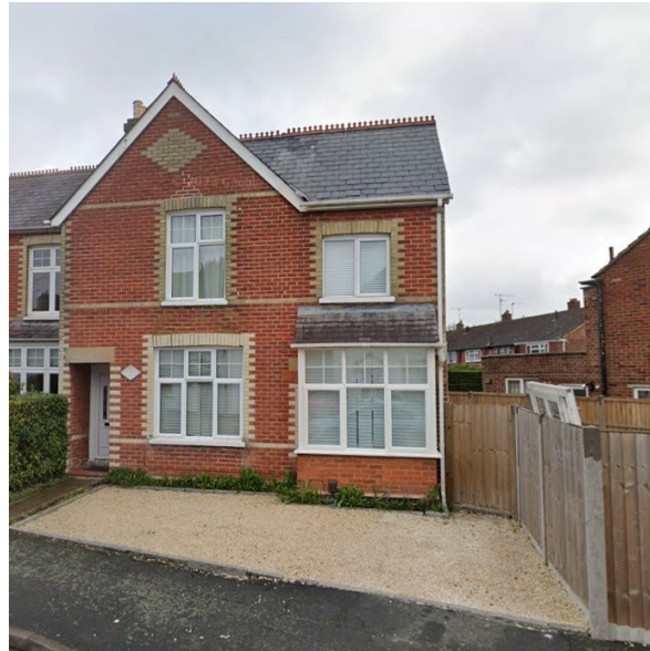
Another example of a double storey side extension with gable roof added to the side
