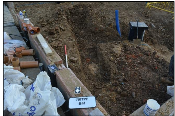
Plate 6: Service 41, view to south
