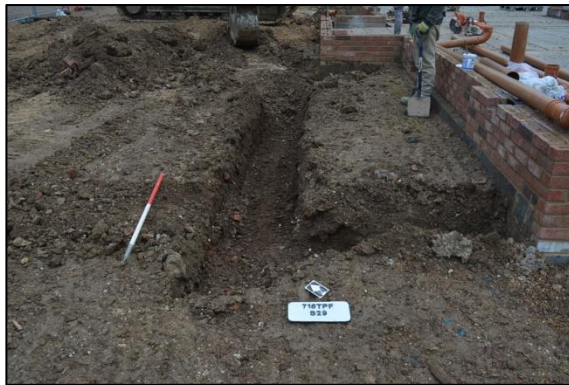
Plate 5: Service 29, view to northeast
