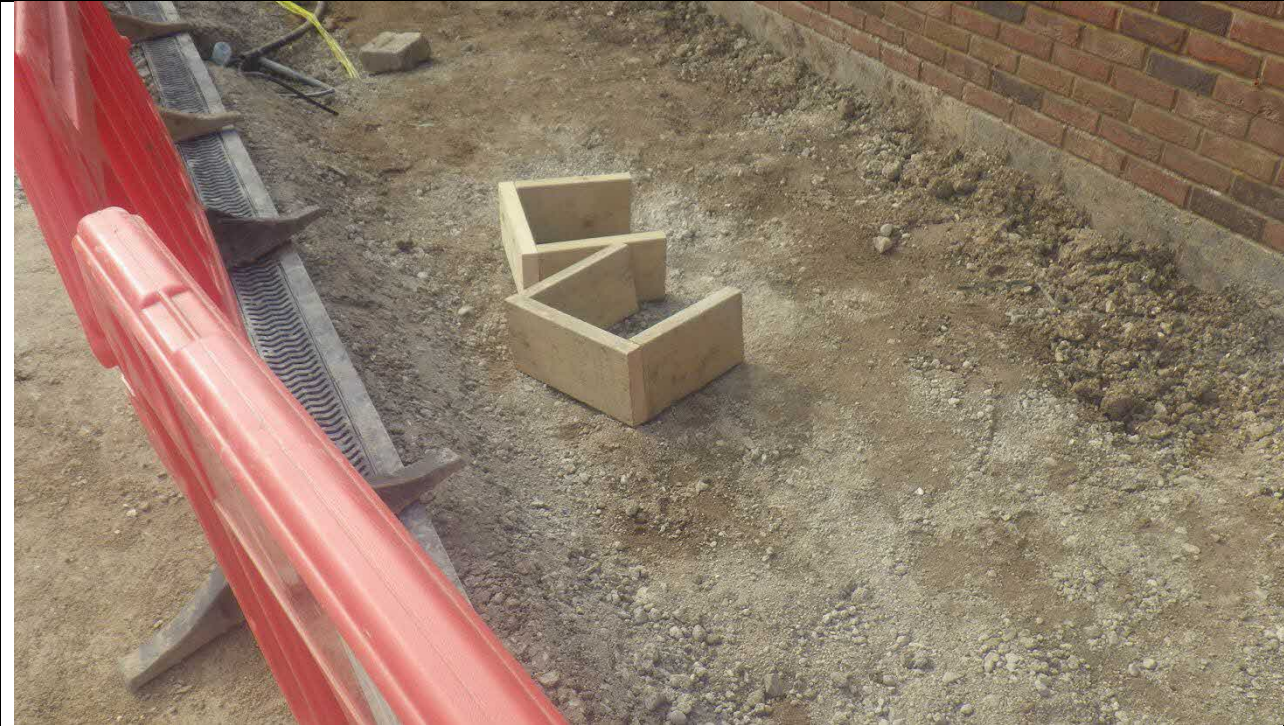
Courtyard area border ready for topsoil
