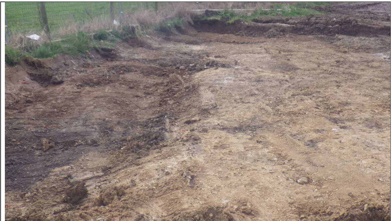
Reduced level dig Plot 1
