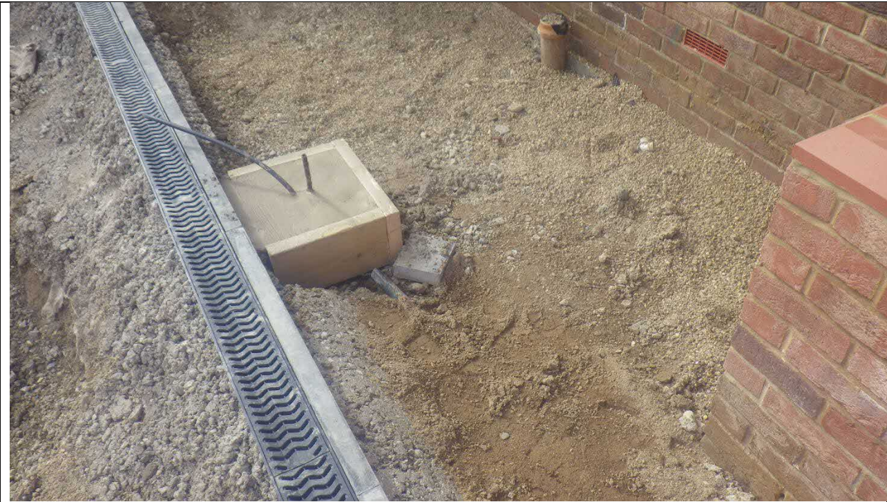
Courtyard area border ready for topsoil
