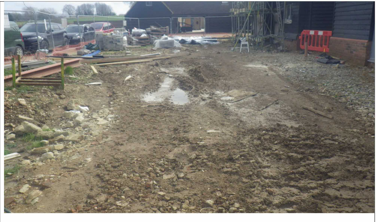
General view east of buildings
