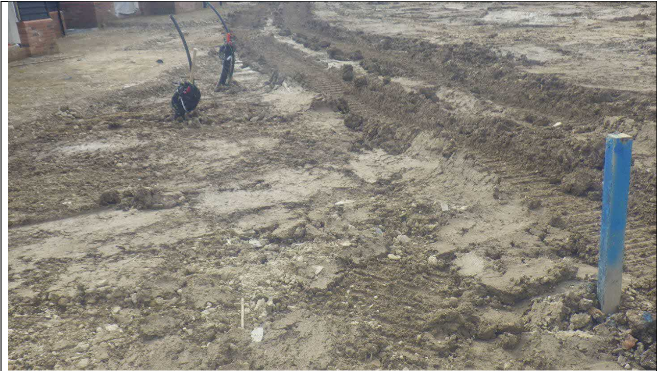
General view north of buildings
