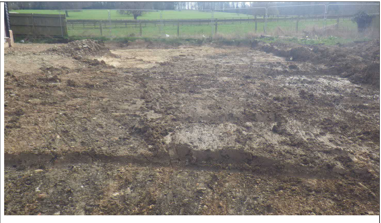
Reduced dig plot 1 garden looking south
