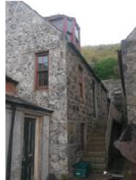
Fig 13 – 2 Storey, Former Access to 1st Floor
