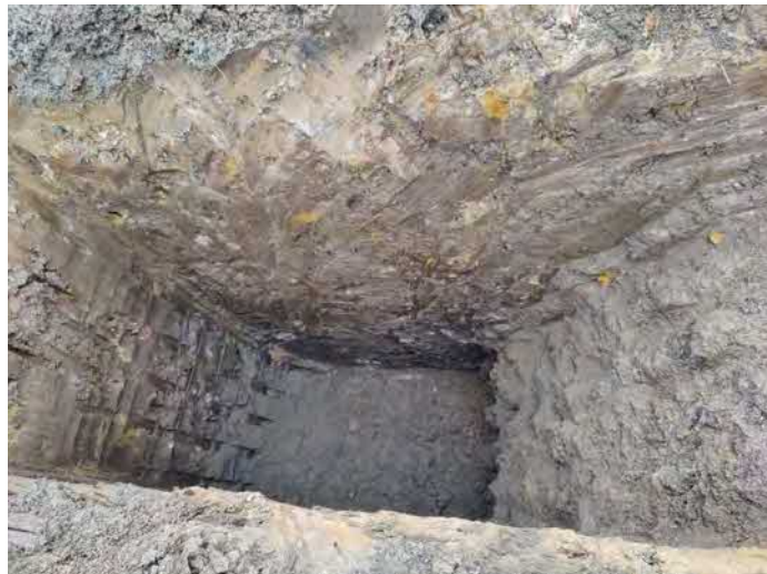
Plate 5 –Cement cap poured into excavation
