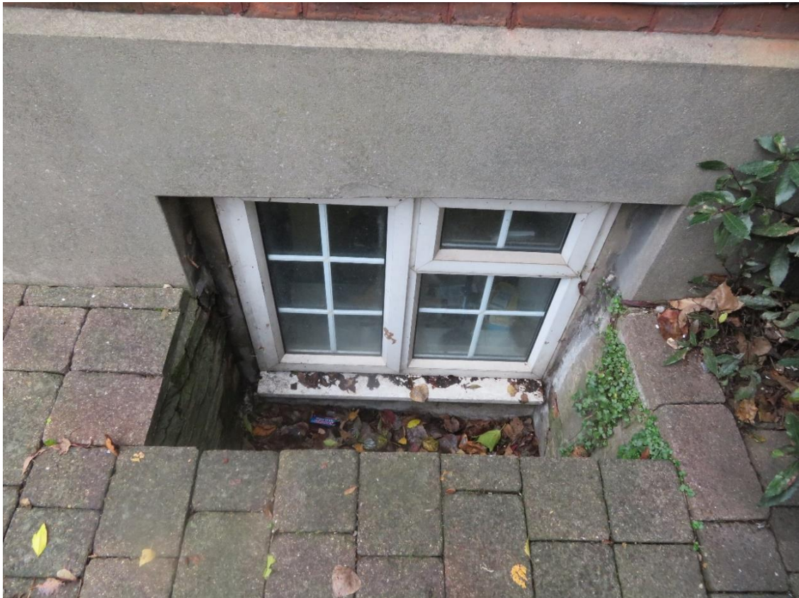
Exterior view of the north cellar window
