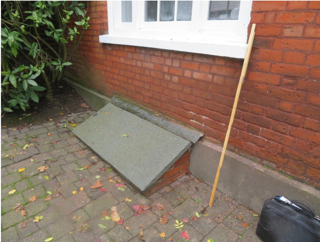
Exterior view of coal chute
