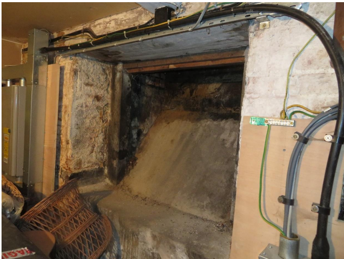
Coal chute in south cellar
