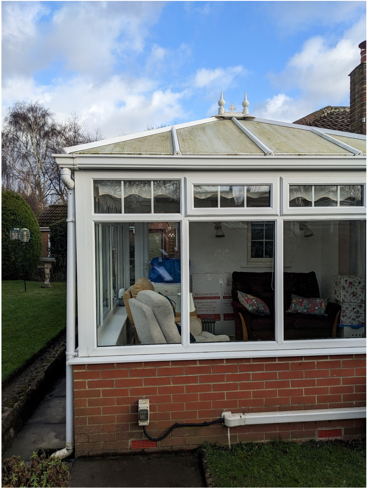
Modern Conservatory to Side/ Rear
