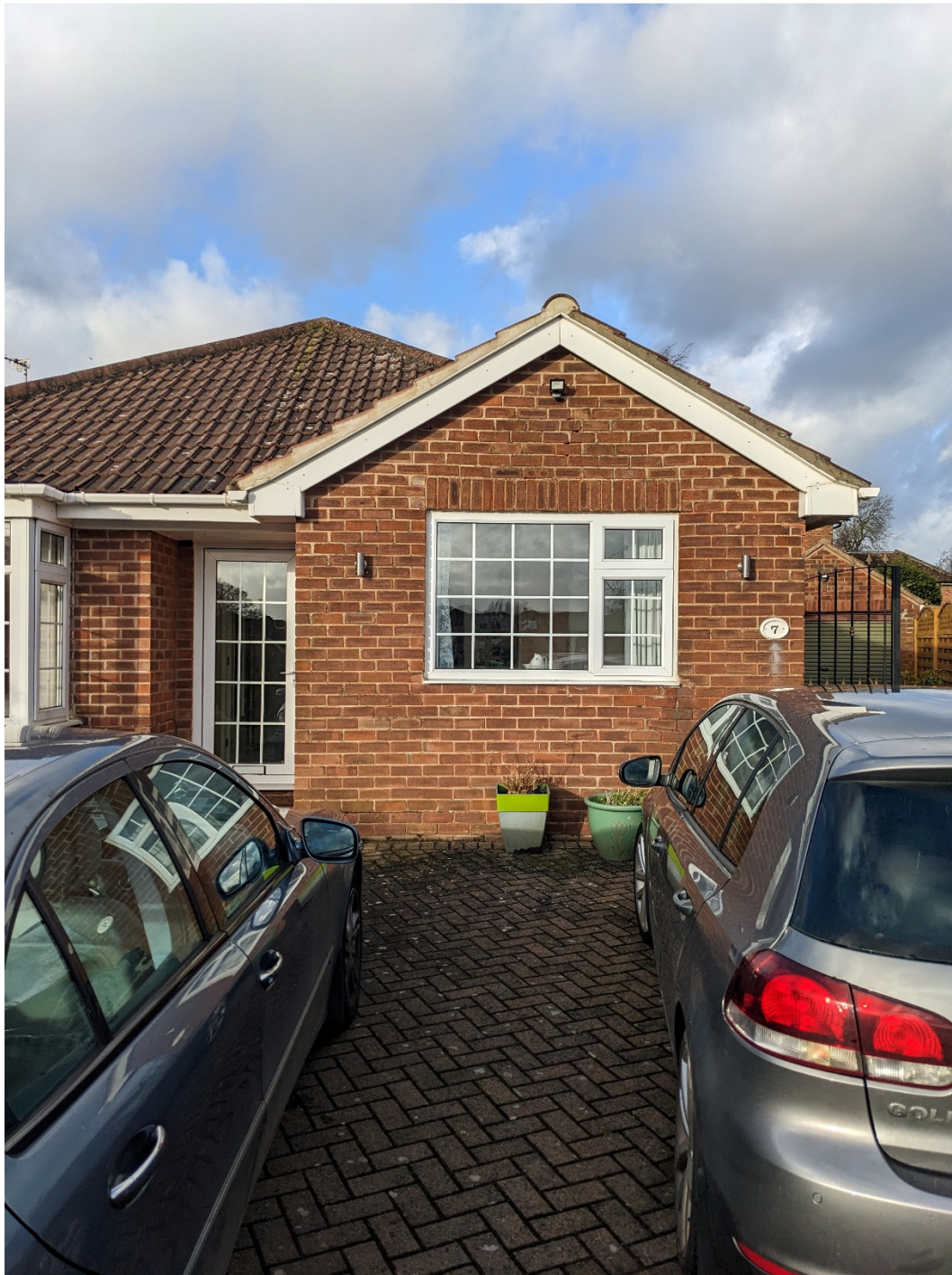
Frontage Showing Modern Roof & Materials
