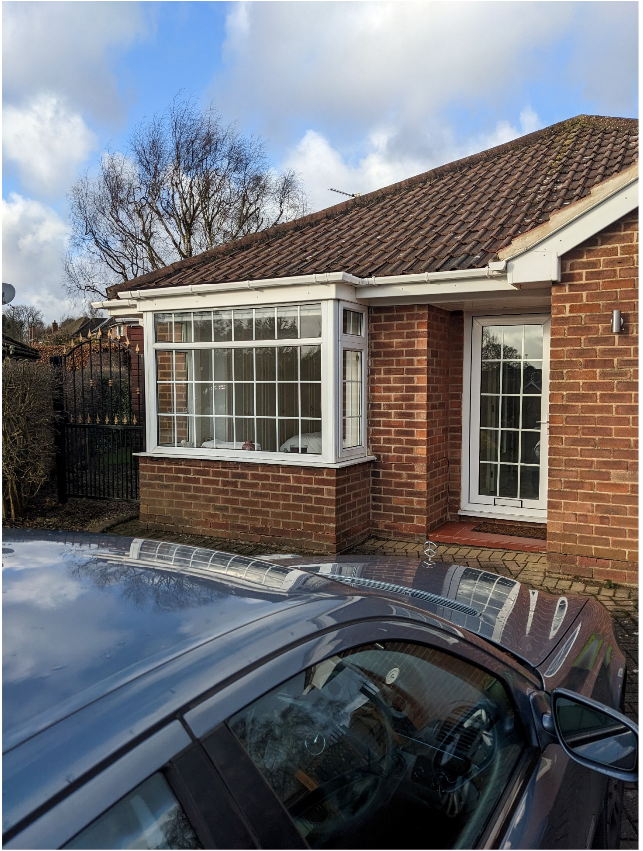
Front External Corner Showing Modern Windows & Sealed Eaves
