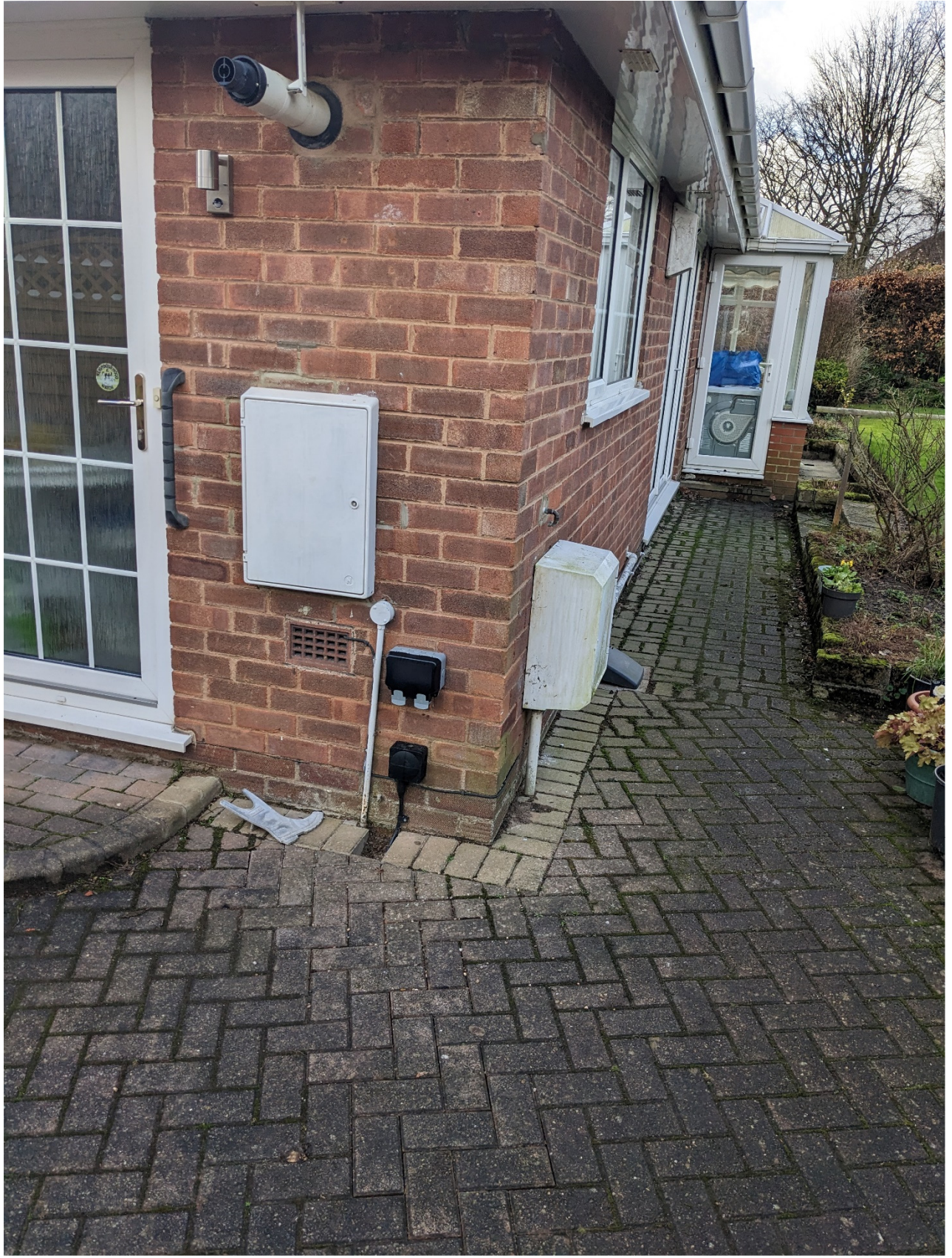
Rear Corner Elevation Showing Sealed Eaves & Modern Detailing
