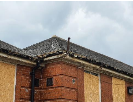
Figure 6 Exposed hipped ridge.
