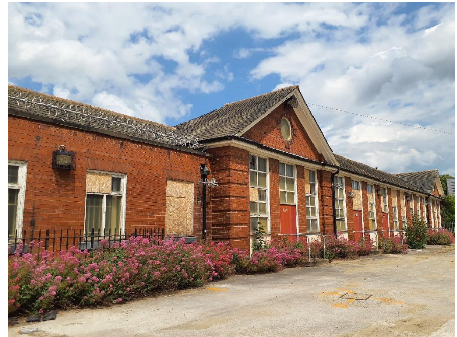
Figure 3 General view of building.
