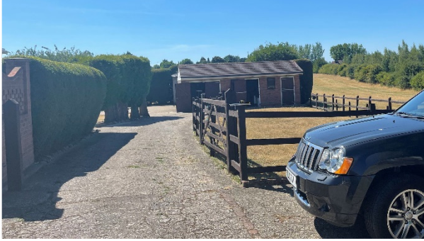
Existing detached outbuilding
