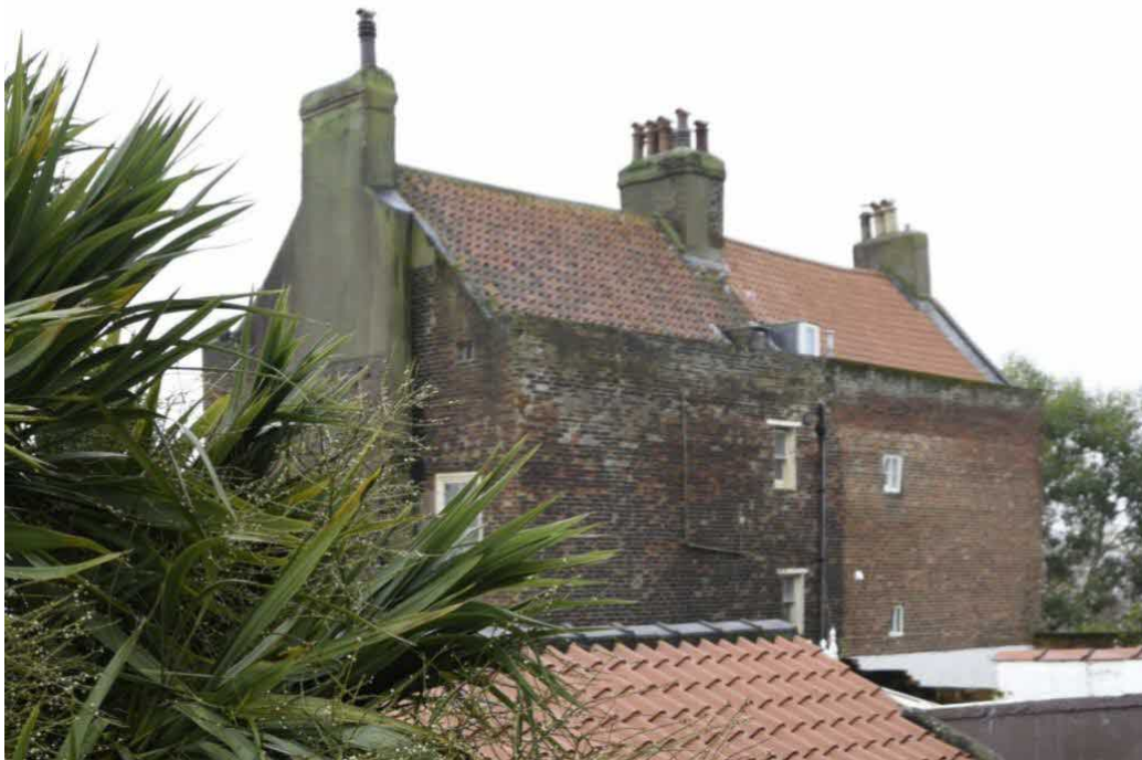
Figure 8, Rear façade of Nos. 32 (right) and 34 (left)
