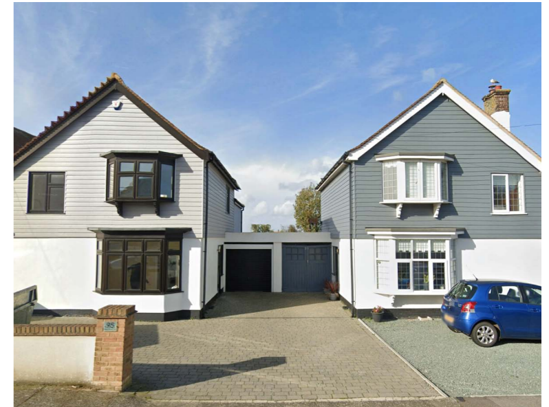
Render and weatherboarding on properties down Percy Ave.
