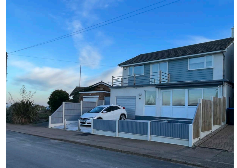
Render and weatherboarding on adjacent property
