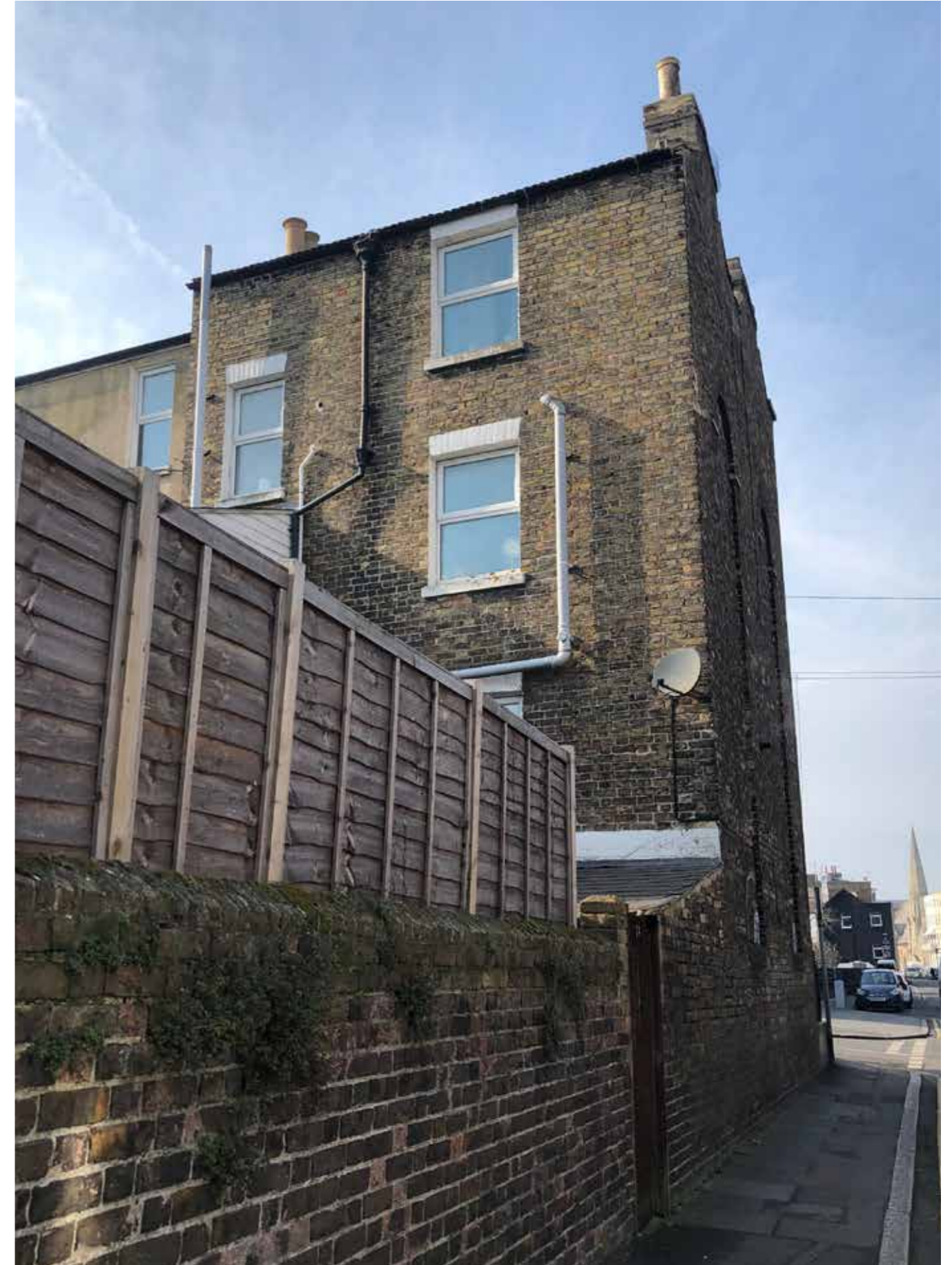
Boundary wall and rear of house from Addington Road
