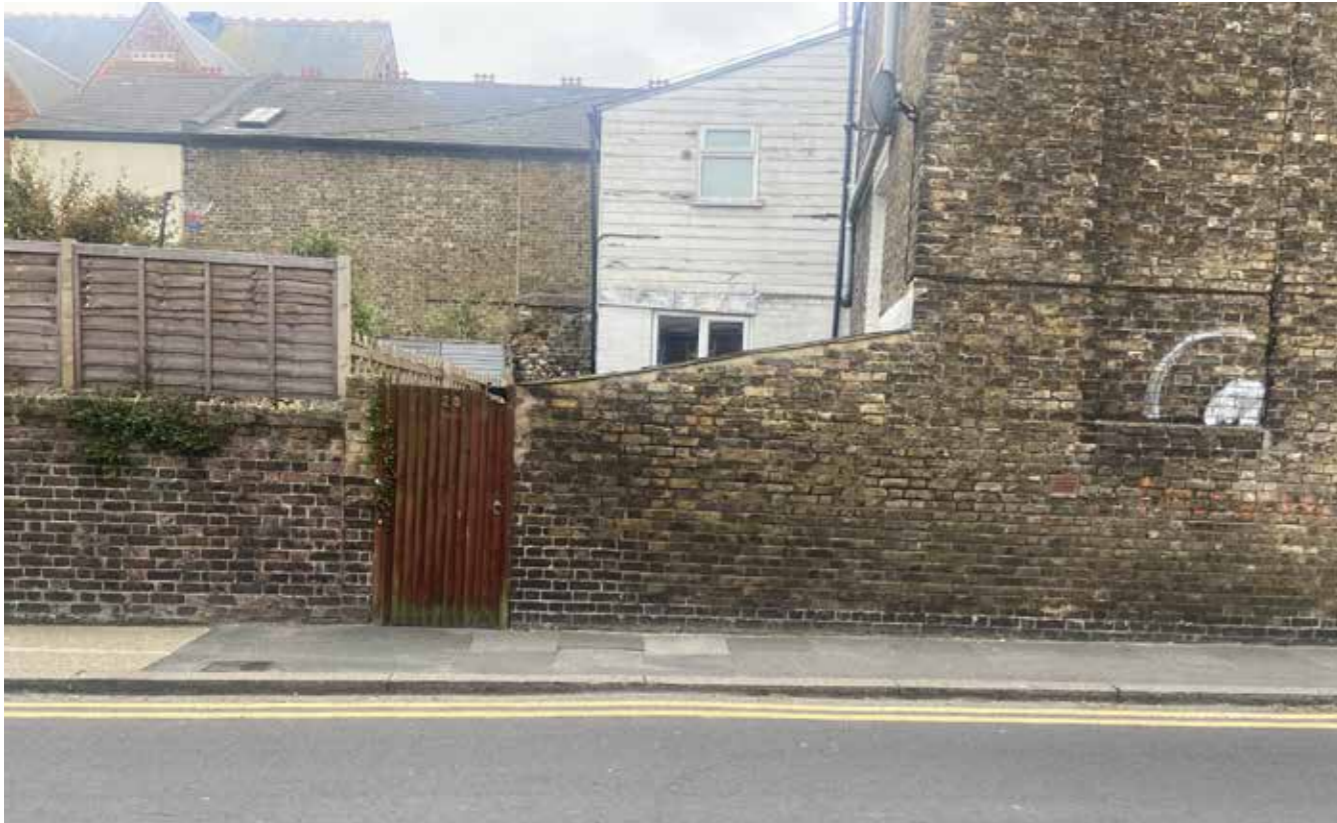
Existing side gate and boundary wall
