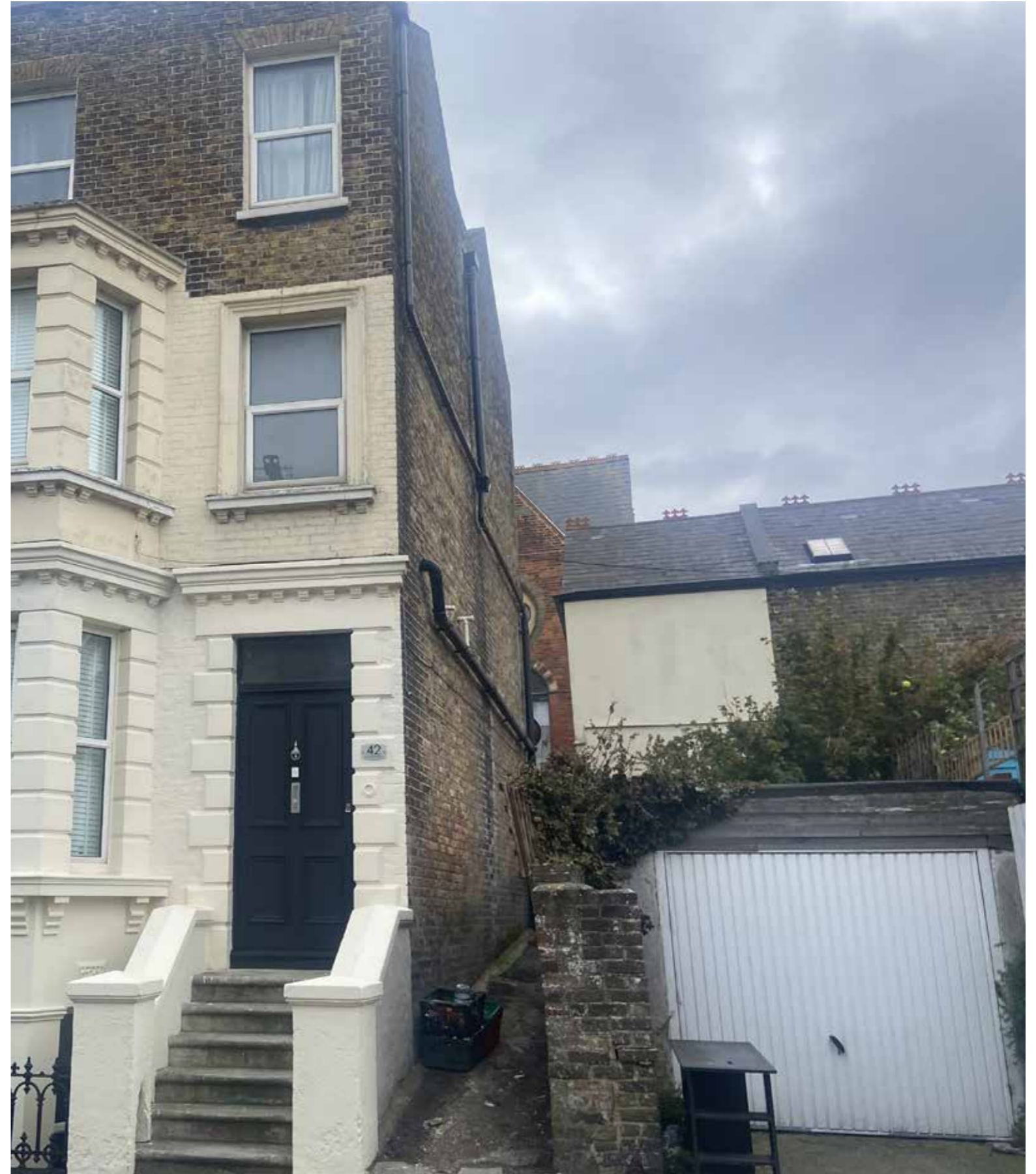
Garage, side alley & 42 Addington Road
