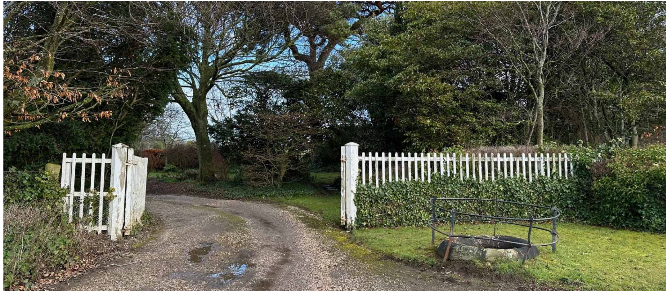
EXISTING ENTRANCE GATE TO BE REMOVED
