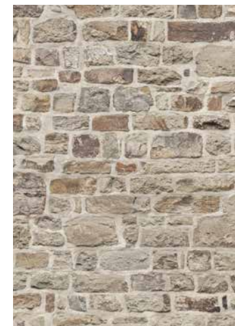
Stonework to match existing
