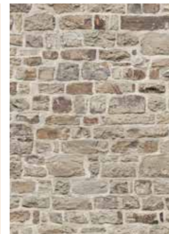
Stonework to match existing
