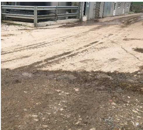
Photograph 6. Existing compacted gravel and concrete hardstanding
