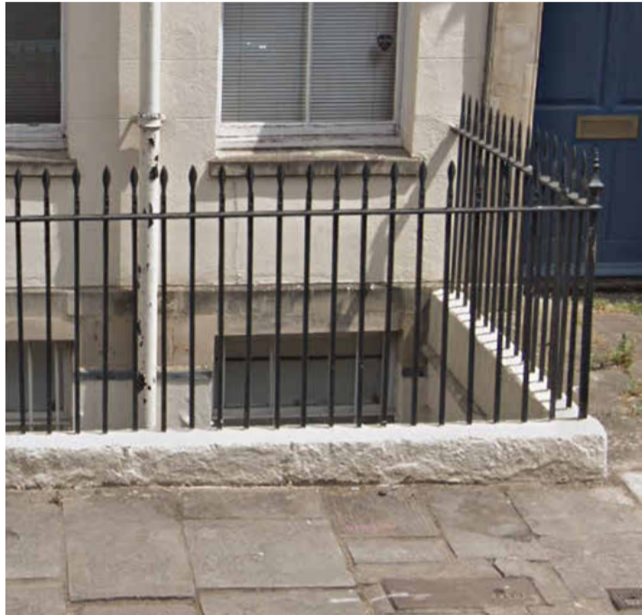
Railings: Current condition July 2019
