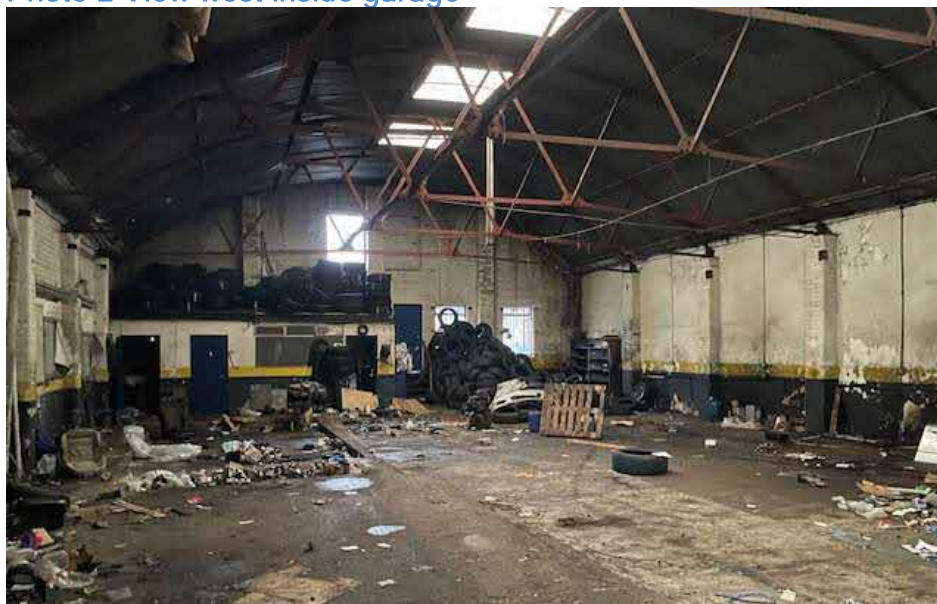
Photo 2 View west inside garage
