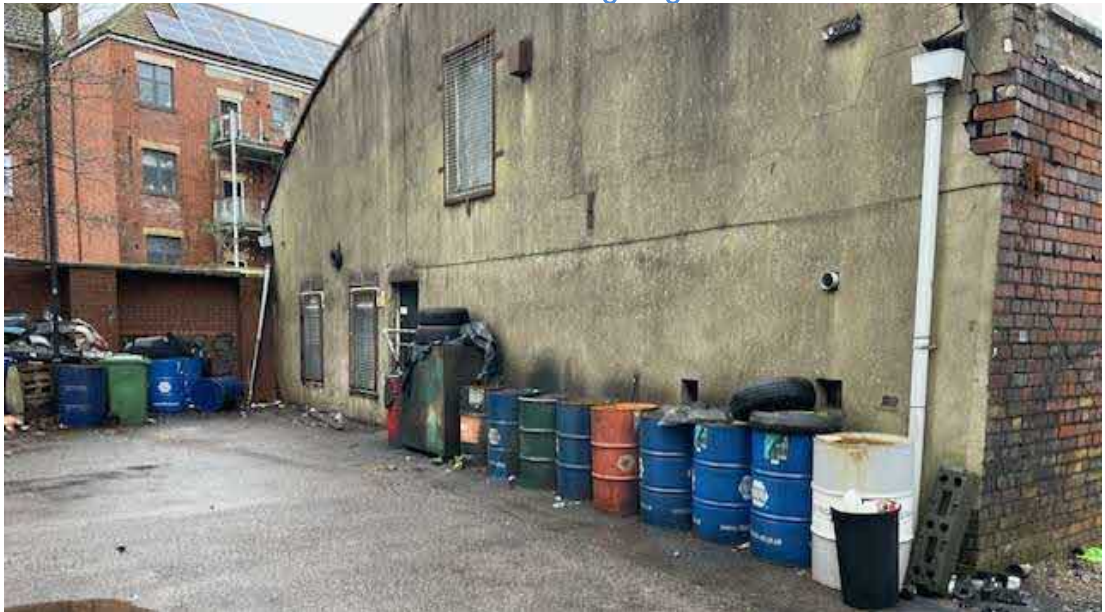
Photo 4 View east of south-western end of garage
