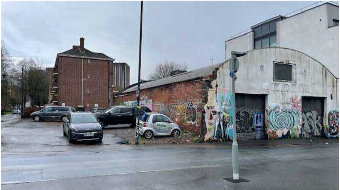
Photo 3 View west of site
