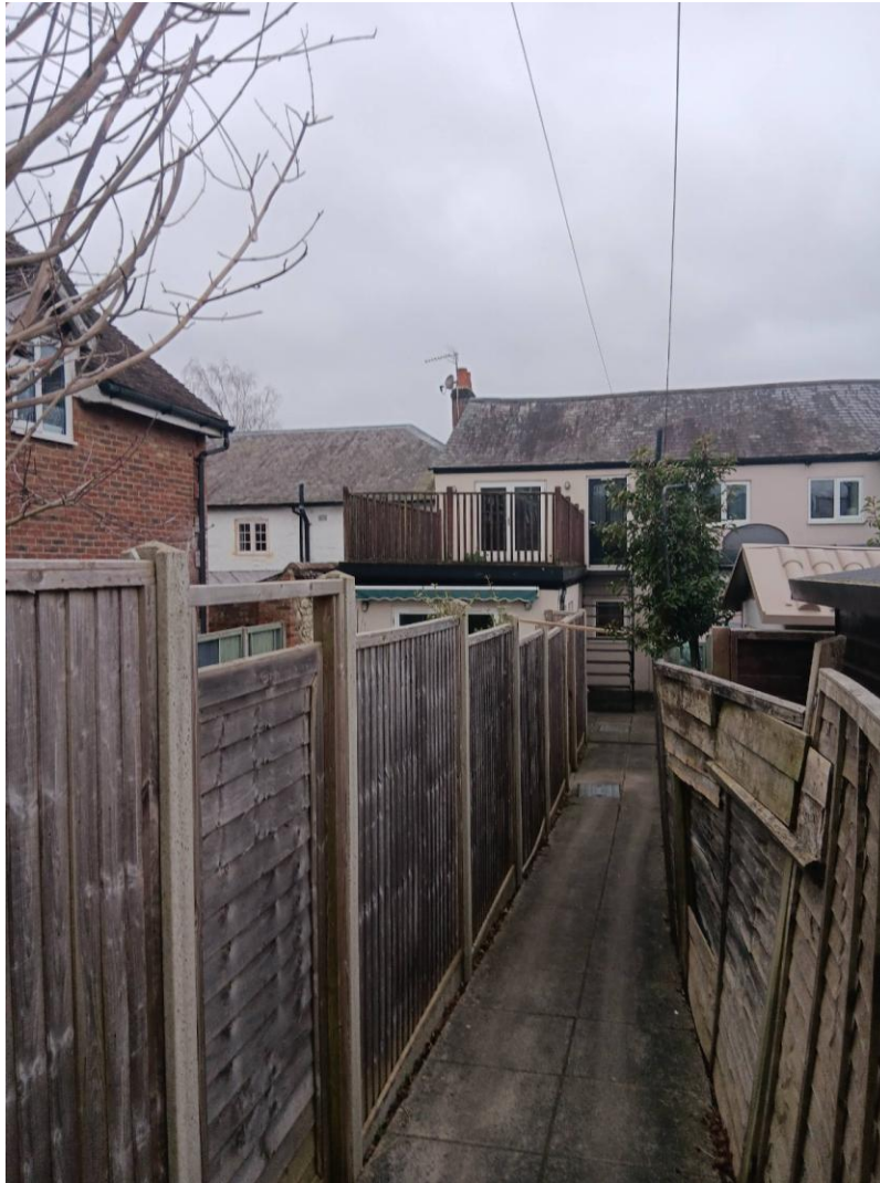
VIEW OF THE REAR OF No 42 & 42A NORMANDY STREET
