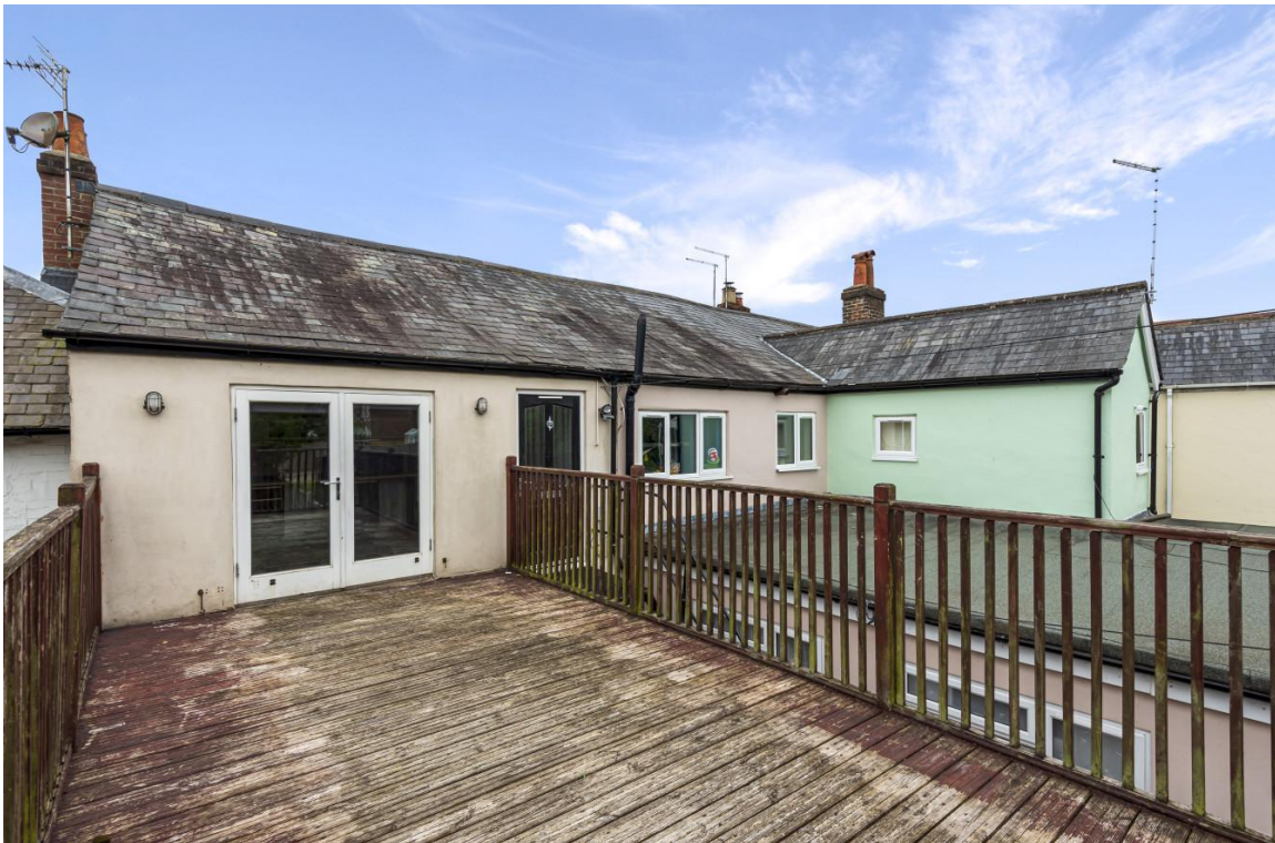
VIEW OF ROOF TERRACE
