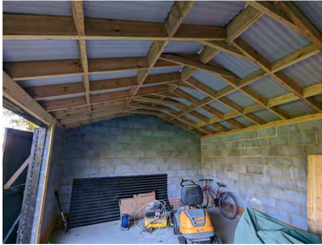
Figure 9. View of the internals of the barn (taken Nov, 22).
