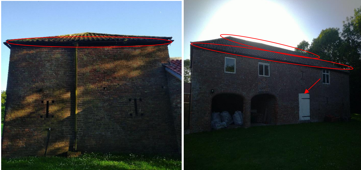
Plate 4.1 – (L) North elevation, (R) – East elevation. Highlighting potential access/roosting points.
