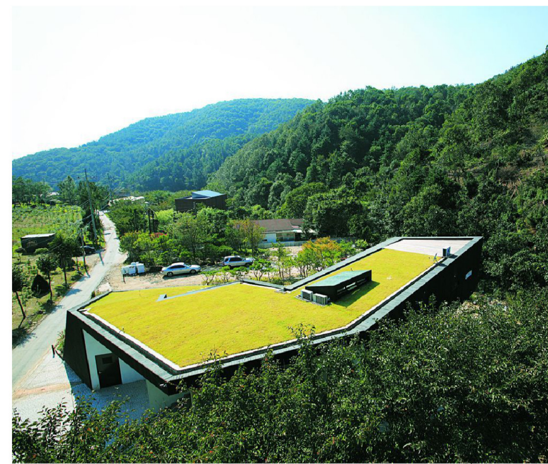
Flat Roof Sedum
