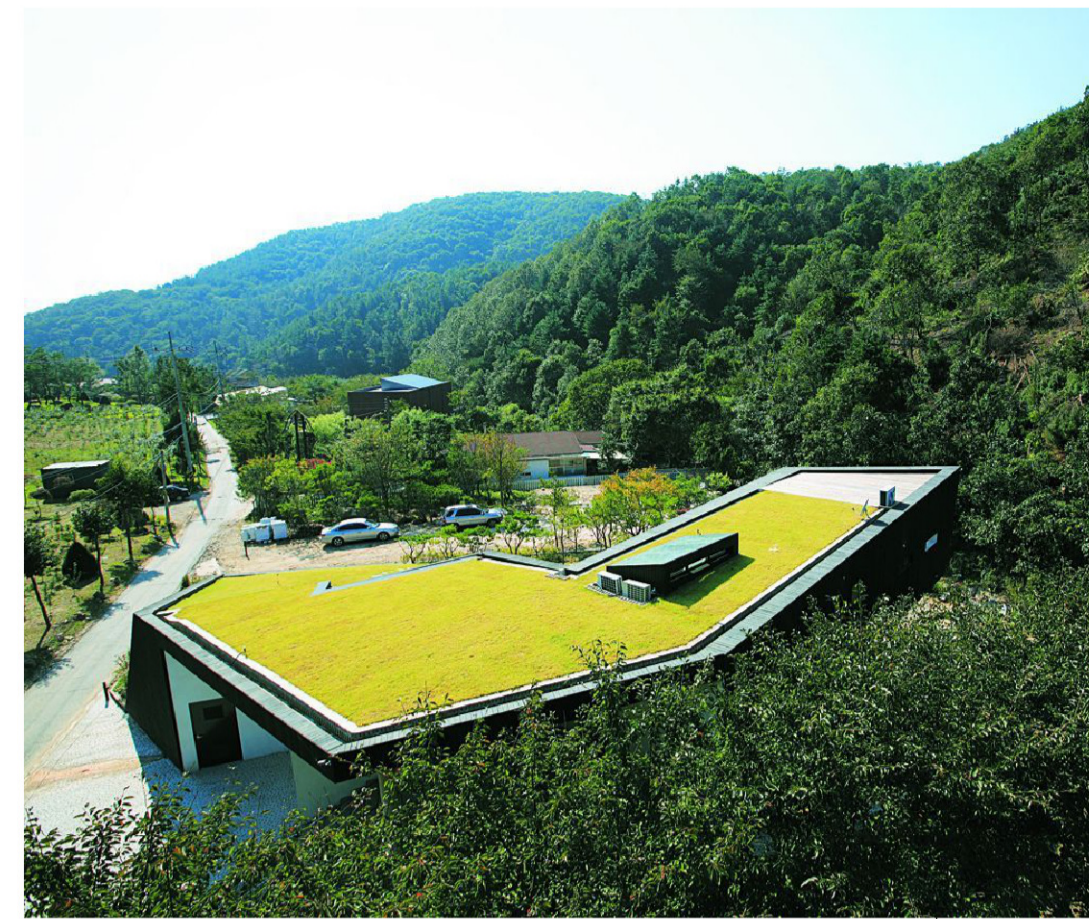
Flat Roof Sedum
