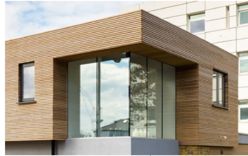
Cedar Cladding western Red Cedar Cladding Battens 19x38mm Vertical
