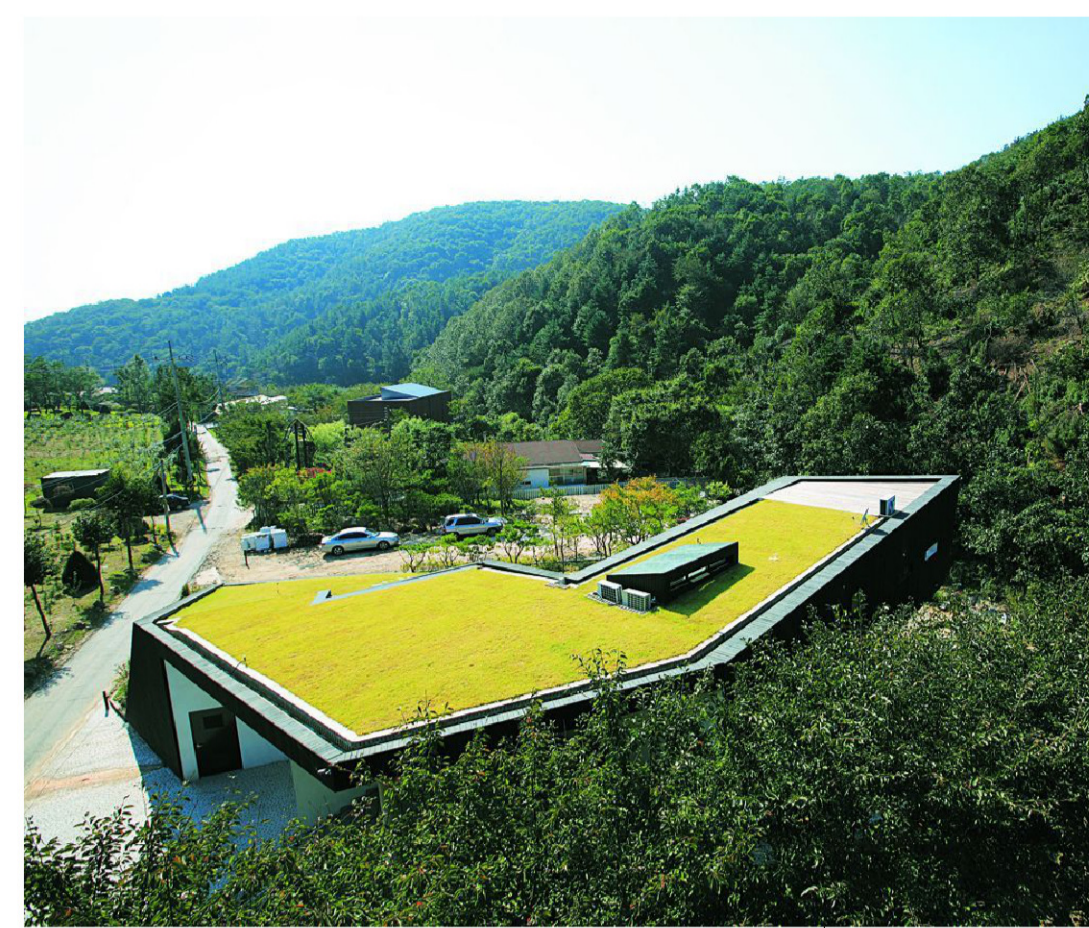
Flat Roof Sedum
