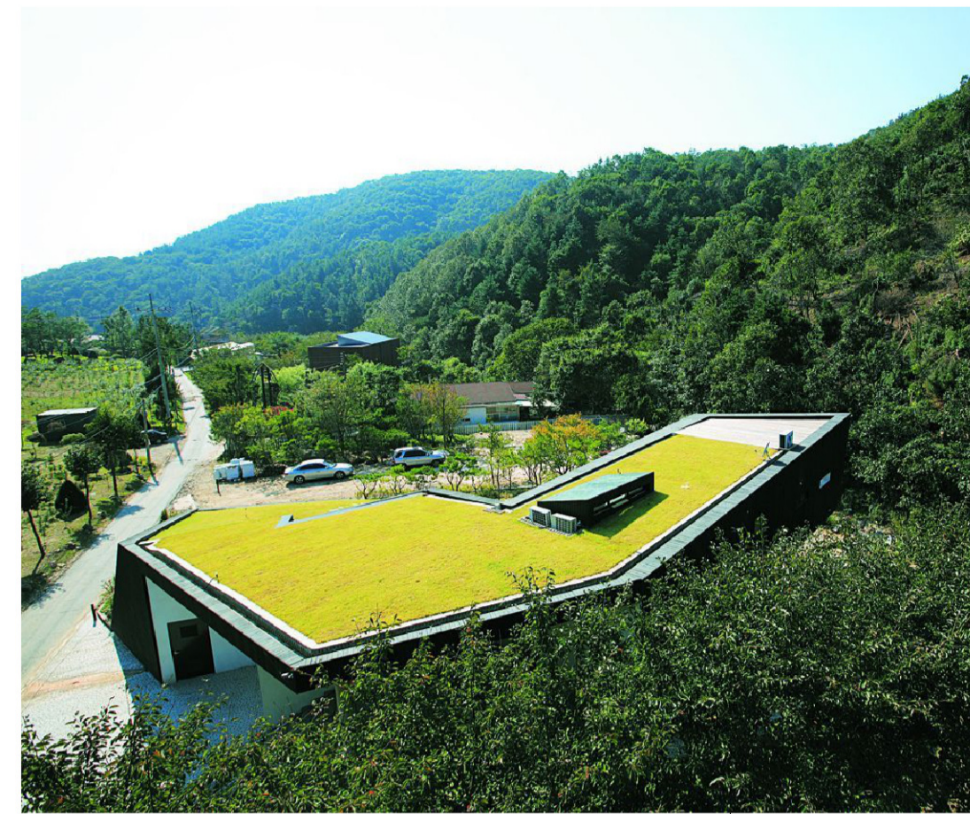
Flat Roof Sedum
