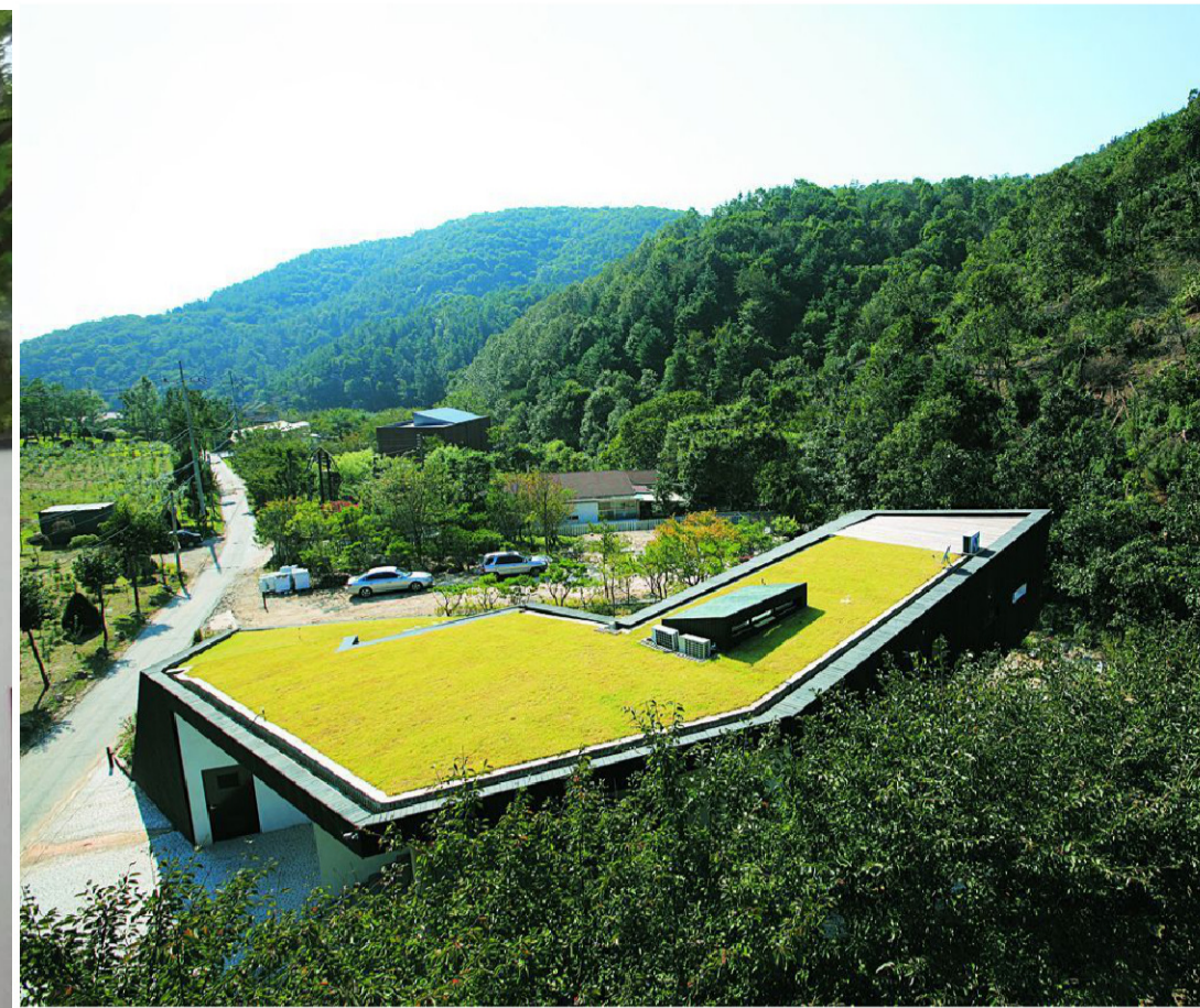
Flat roof - Sedum Roof
