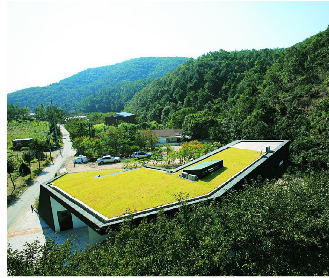
Flat roof - Sedum Roof
