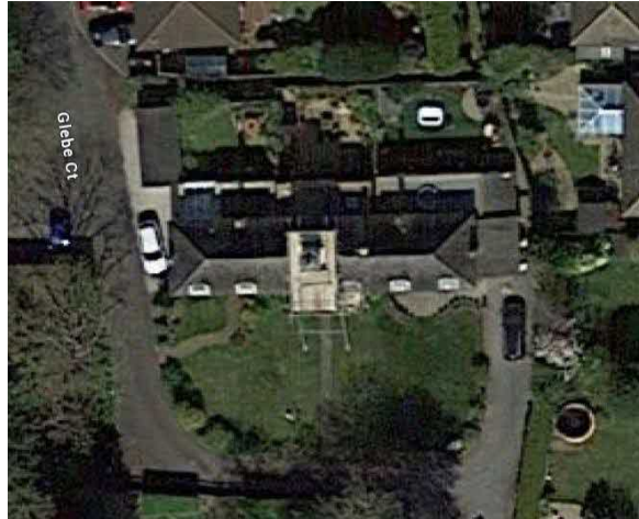
Figure 1: Aerial view of 1-3 The Clock House, Glebe Court
