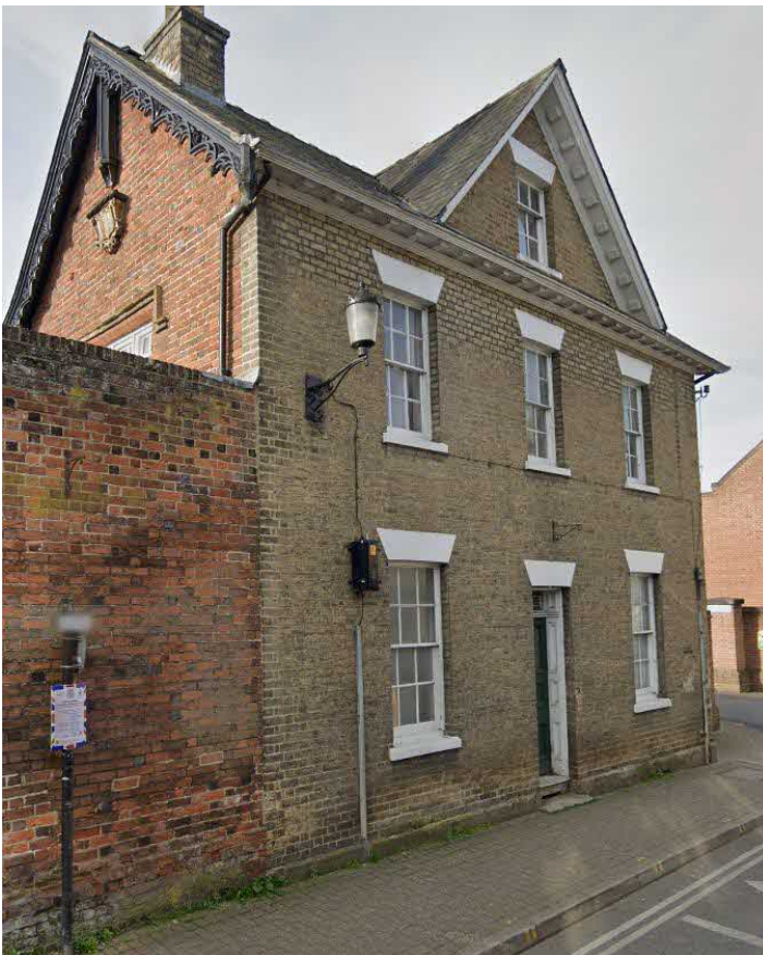
North and East elevations from Hill Street.
