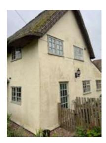
It is proposed to replace the circa 1960/70's side door, frame and threshold to the house with a solid hardwood stable door style door with glazing in the top half. Frame and threshold will also be hardwood. This door is located on the North side of the property within the circa 1960 extension to the front of the property.
