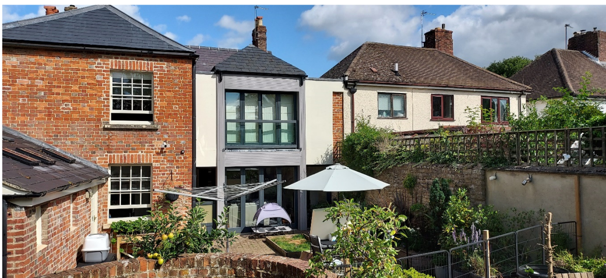
Photo showing 2002 2-storey extension with service range on left and C20 house on right
