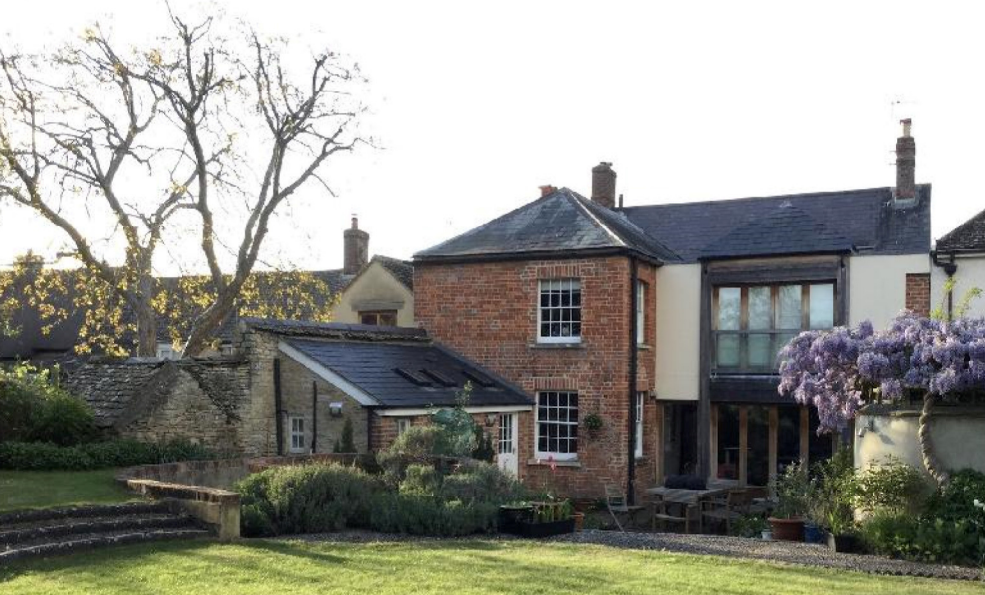
Rear elevation with existing lean-to rear wing against stone wall boundary
