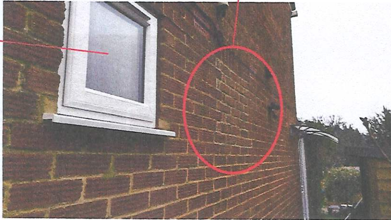
Existing wall, showing downstairs toilet window to the left, and new brickwork (circled) where the original window was formerly located
