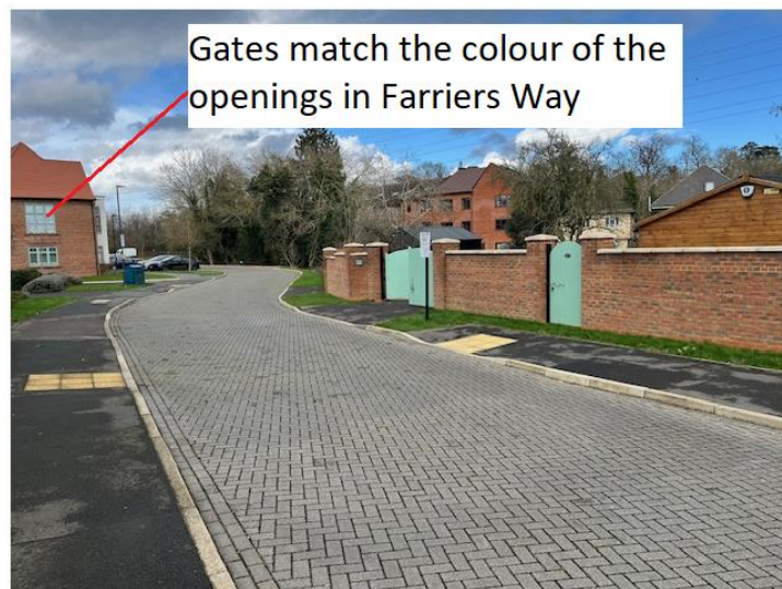
Photographs of the boundary wall, gates, and fence
