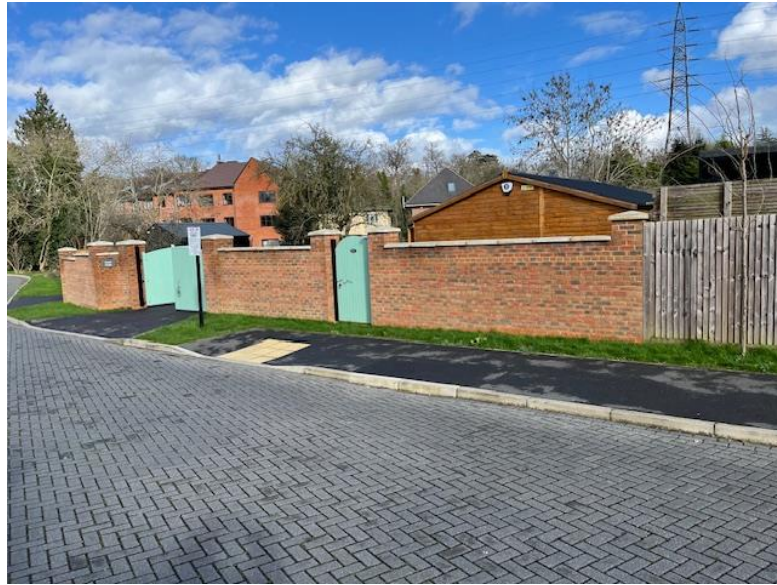
Boundary wall and gates
