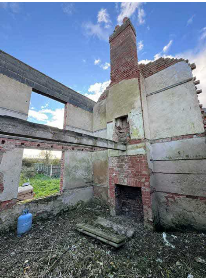
GENERAL VIEW WITHIN NORTH EAST ROOM – LOOKING SOUTH
