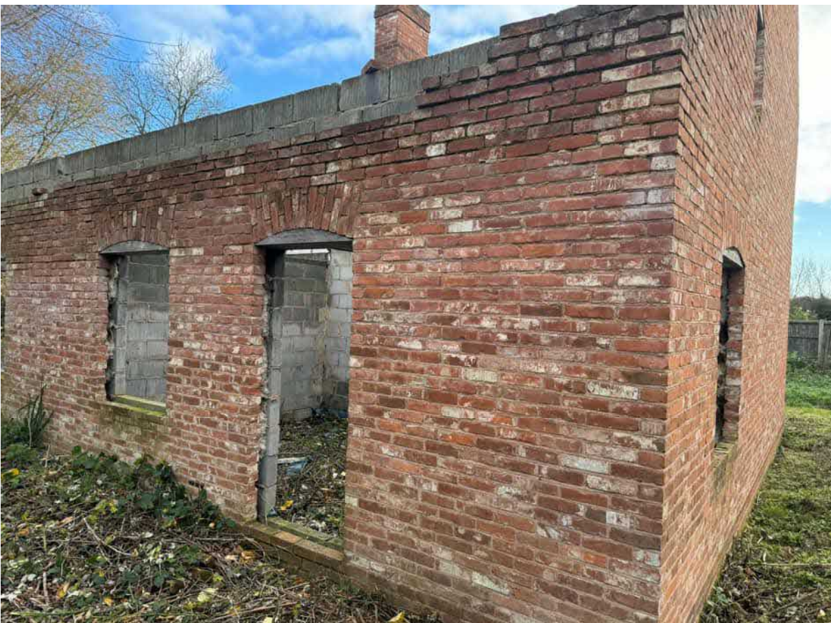
NORTH WEST ELEVATION – REAR – LOOKING EAST
