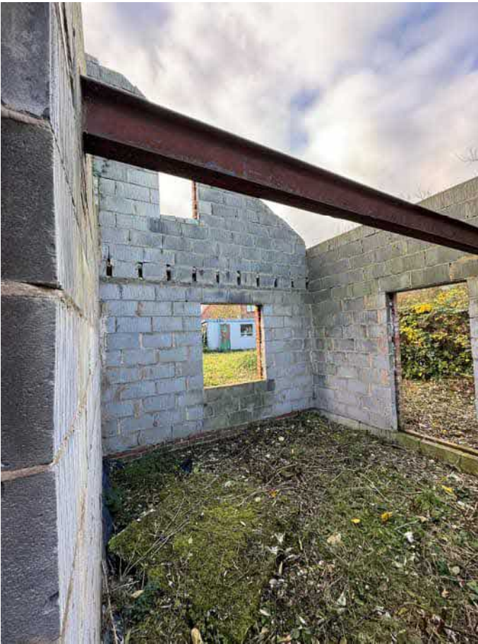
GENERAL VIEW WITHIN SOUTH WEST ROOM – LOOKING SOUTH
