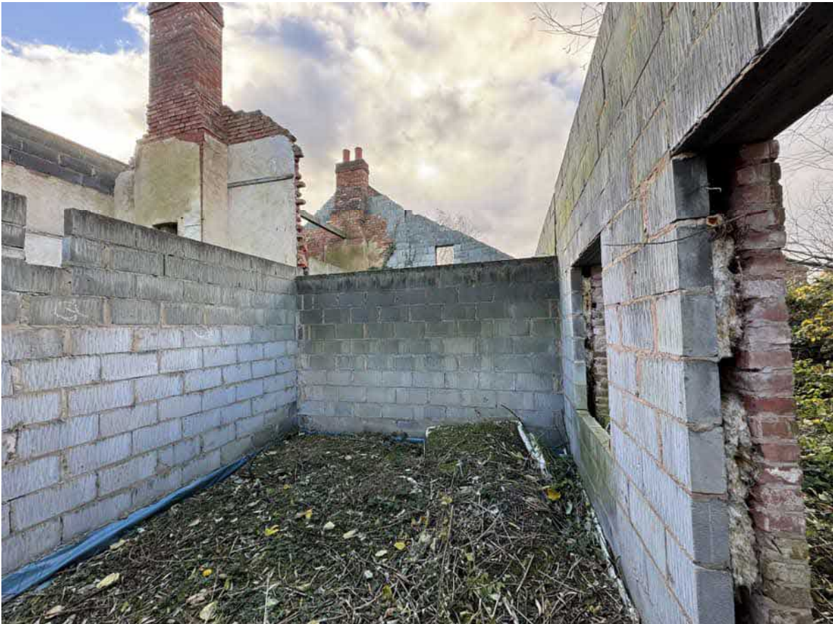
GENERAL VIEW WITHIN NORTH WEST ROOM – LOOKING SOUTH
