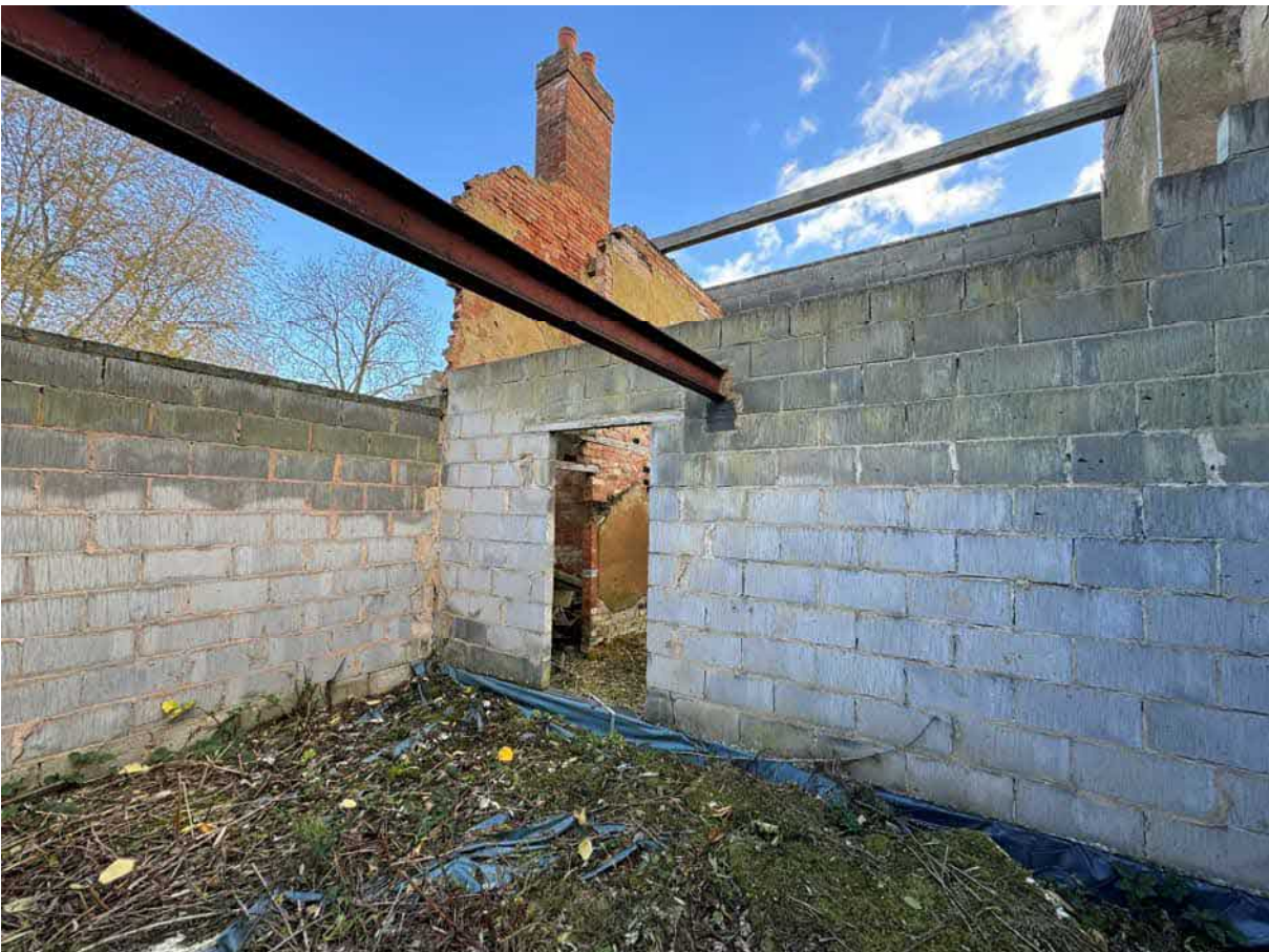
GENERAL VIEW WITHIN SOUTH WEST ROOM – LOOKING NORTH-EAST
