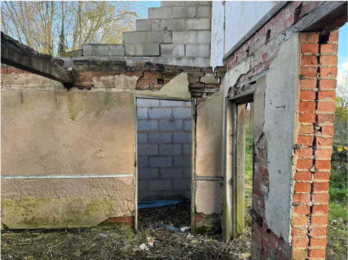
GENERAL VIEW WITHIN NORTH EAST ROOM – LOOKING NORTH
