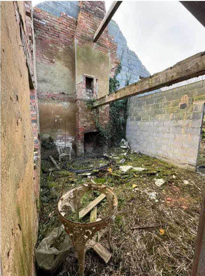
GENERAL VIEW WITHIN SOUTH EAST ROOM – LOOKING SOUTH
