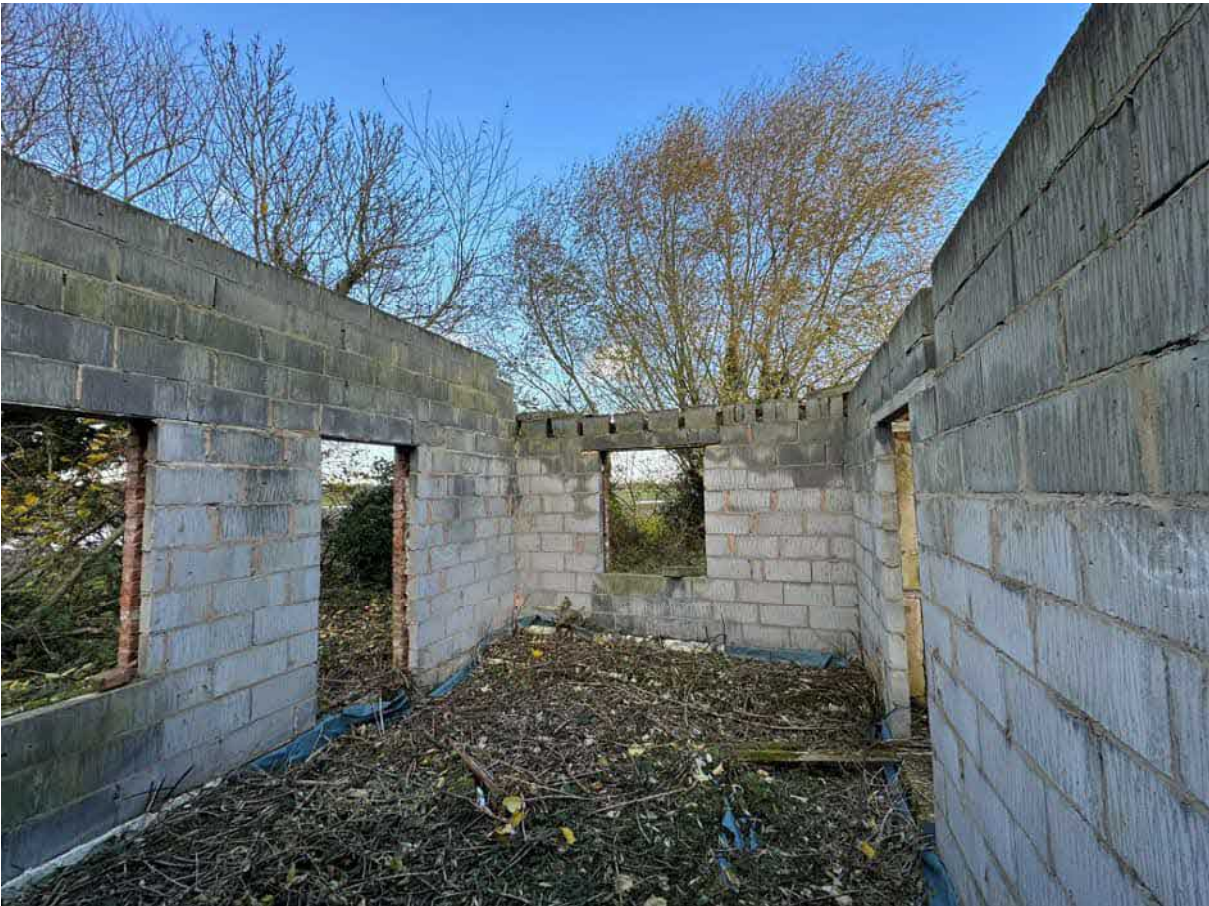
GENERAL VIEW WITHIN NORTH WEST ROOM – LOOKING NORTH
