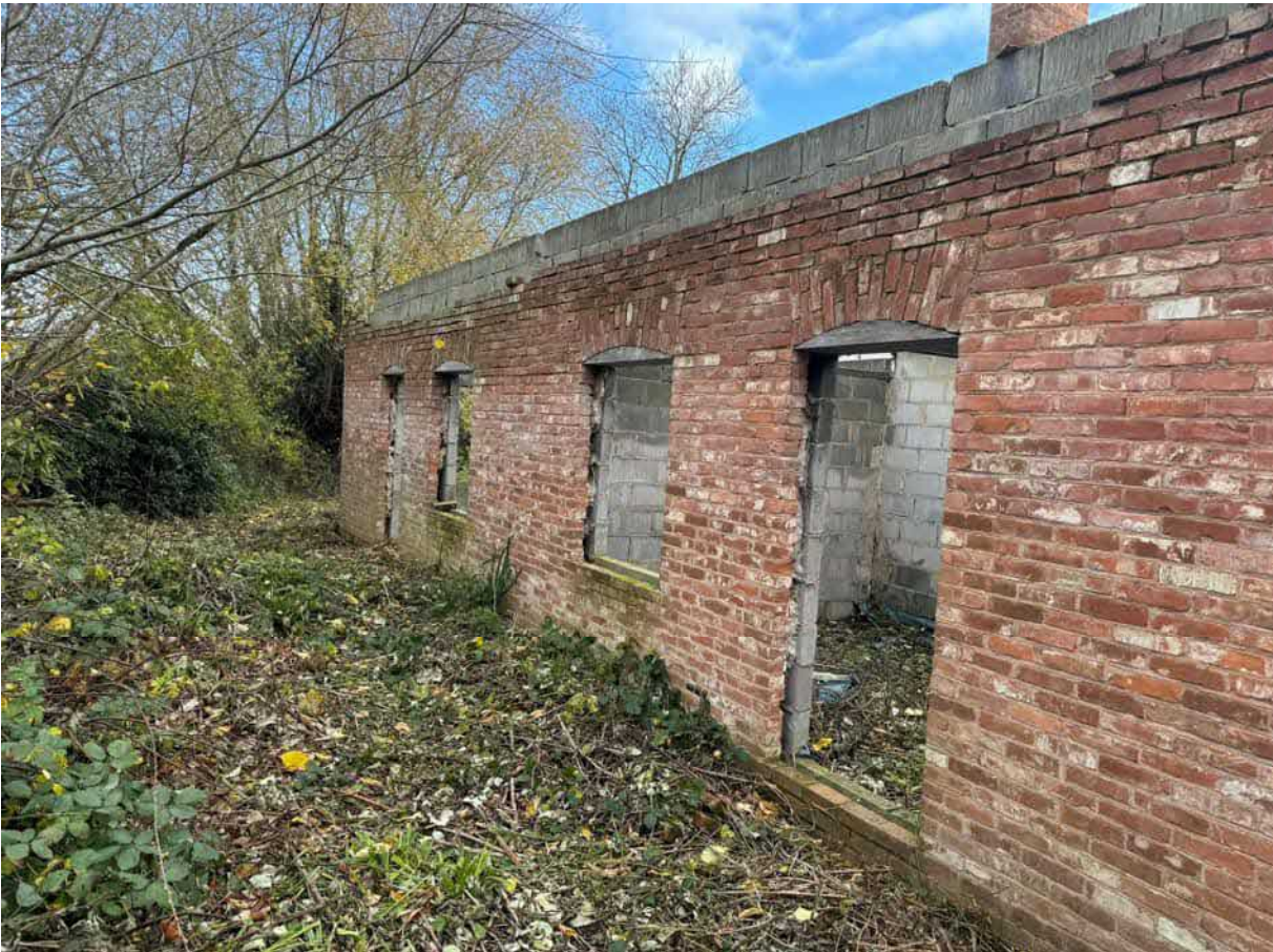
NORTH WEST ELEVATION – REAR – LOOKING NORTH EAST
