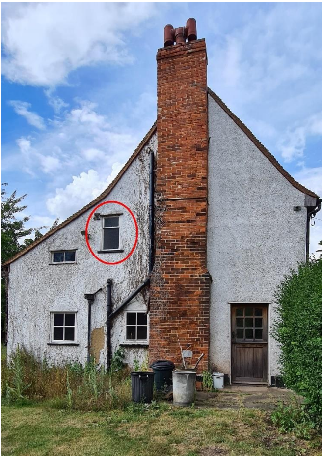
Fig 6. Side elevation (south) mid-20 th century metal framed windows to be replaced.
