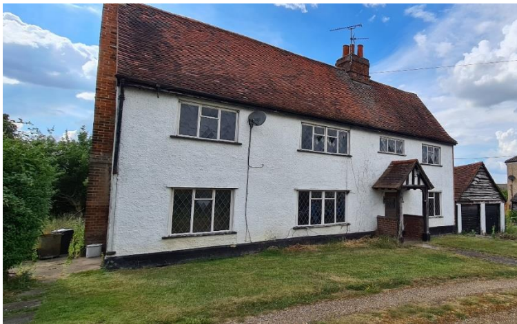
Fig 2. Photograph of the front elevation
