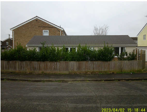
Illustration 1: View of site from street level
