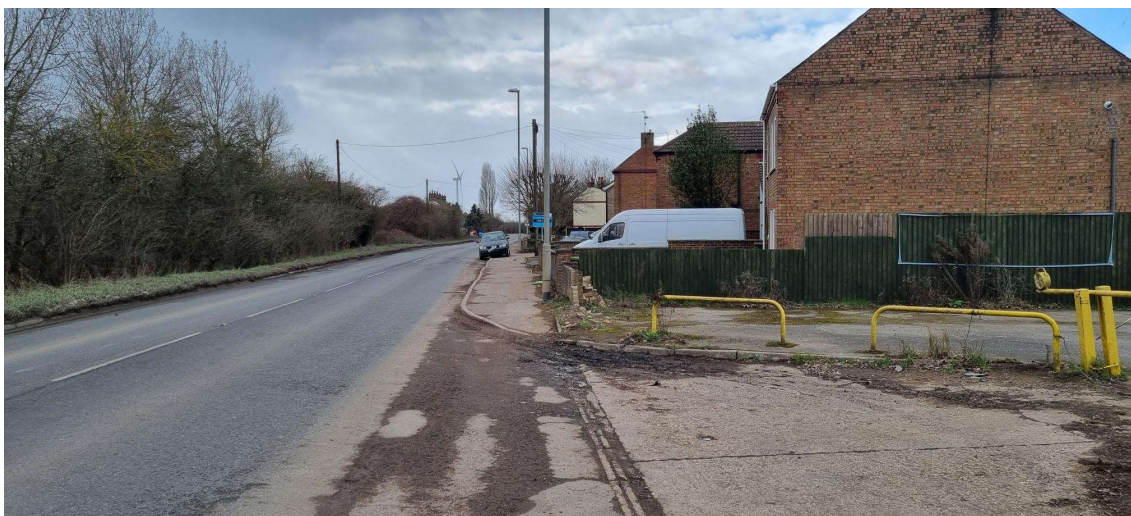
View west along Peterborough Road (photo taken outside of Aster Cars site, centrally along frontage)
