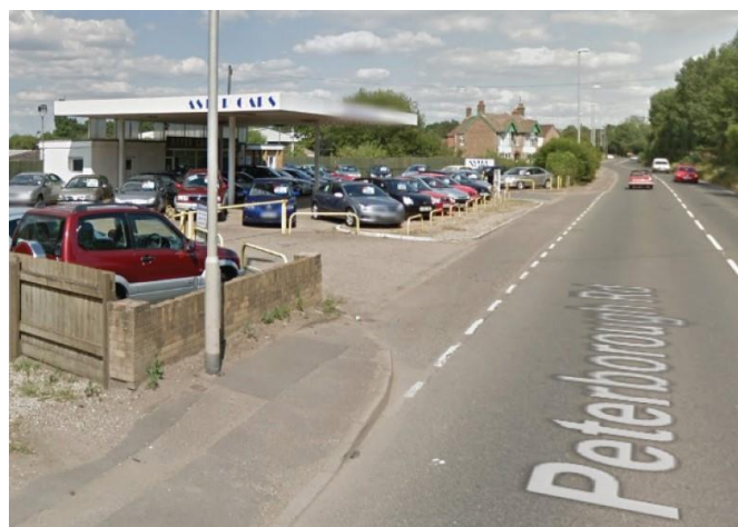
Plate 1 - Existing Gap in Footway Provision along Peterborough Road outside Aster Cars site (image courtesy of Google Streetview)
