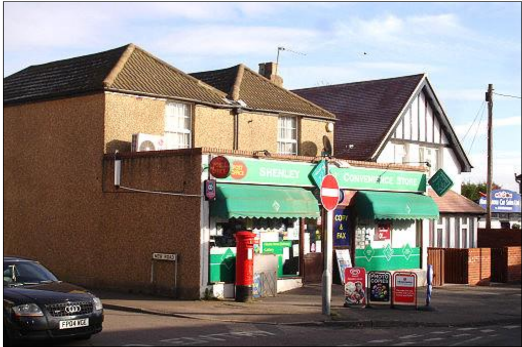
Figure 13. Unattractive shop front
