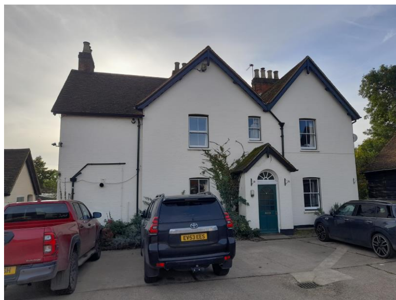
Image 11 Front elevation of Grade II listed Pursley Farmhouse
