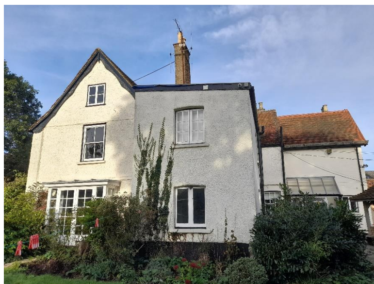
Image 4 View of South East facing elevation, with Bathroom window proposed for replacement under flat roof
