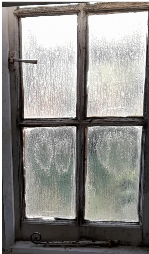
Image 9 Ironmongery will be retained for replacement window
