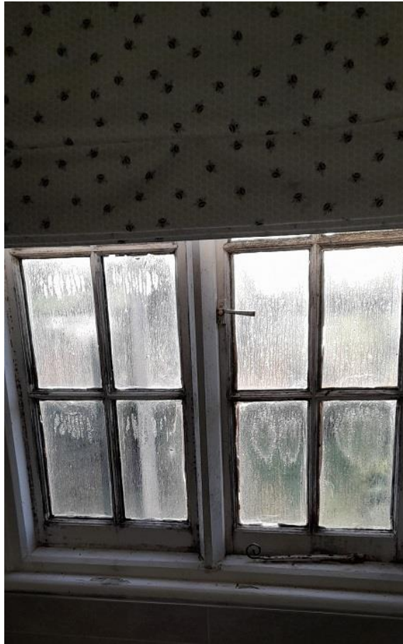
Image 8 Condensation to both casements highlights poor environment within Bathroom
