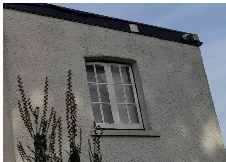
Image 6 External close up of existing Bathroom window
