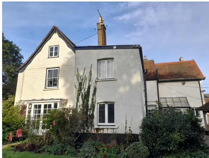
South East elevation of Pursley Farmhouse
