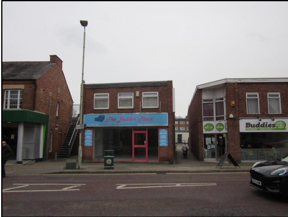
Photograph 1. Existing building, 57 - 59 Leicester Road, Wigston
