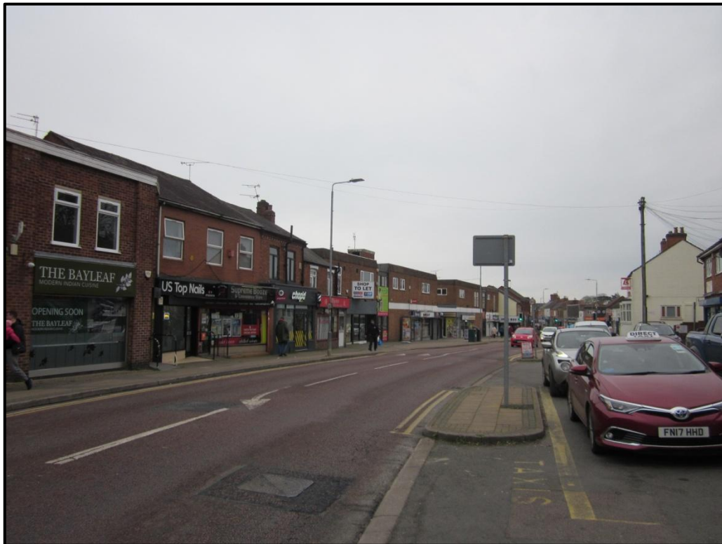
Photograph 3. Commercial premises on Leicester Road to the South of the application site
