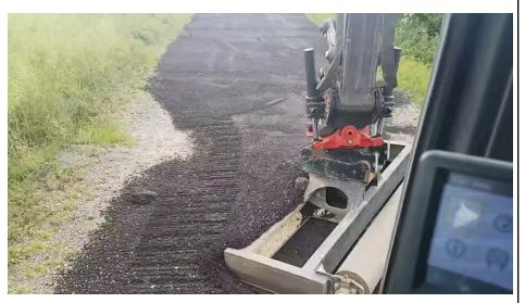
Finally, a top layer of road planings or concrete will cover the hardcore and make a smooth top layer.
