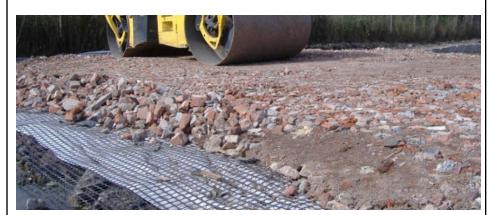
Installation of hardcore (crushed brick) and compaction of the same, the geotex is then used to bind the layers together.
