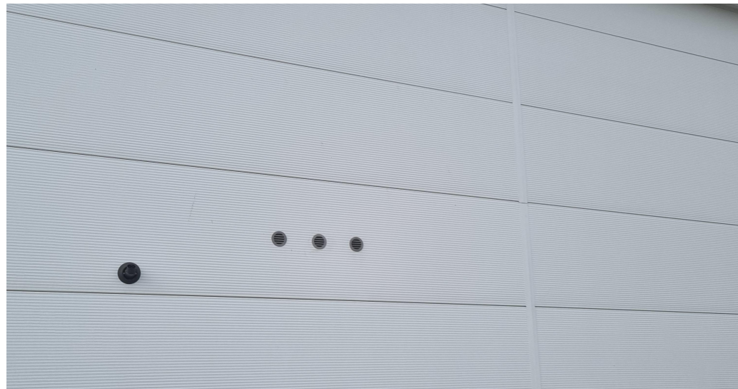
Gable, Front & Rear Wall Cladding (on Show) - Kingspan MR1000 - White
