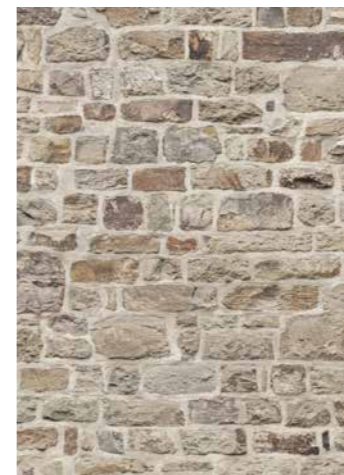
Stonework to match existing
