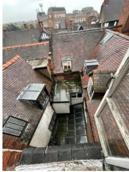
Internal roof scape
