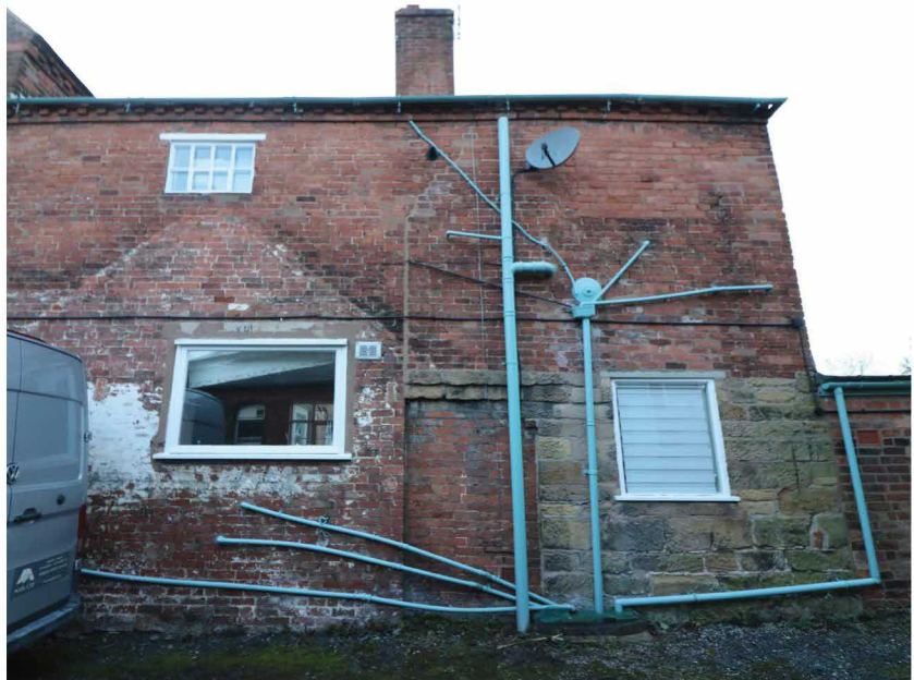
Side of Chestnut House (from east)
