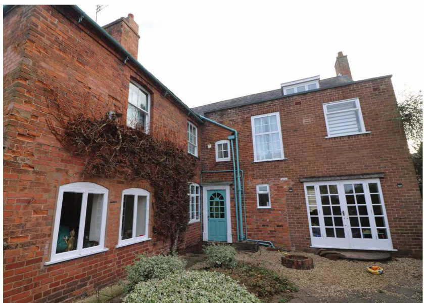
Rear of Chestnut House (from south)
