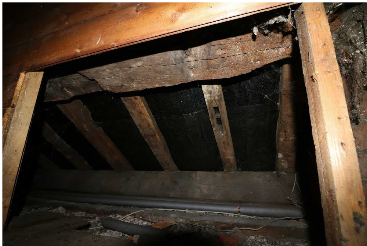
Figure 36 View of roof structure in loft space accessed from room C2
