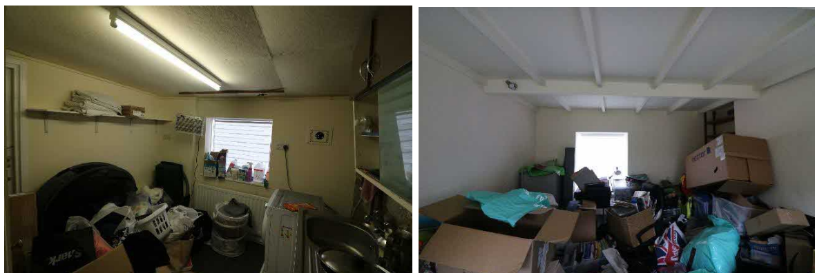
Figure 24 Interior of Rooms A5 (right) and A6 (left)
