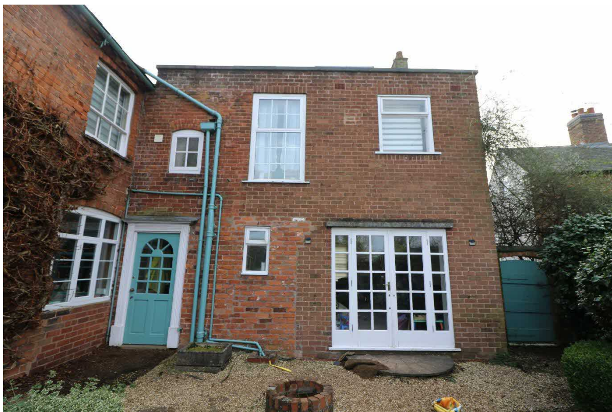
Figure 14 Rear (southern) elevation
