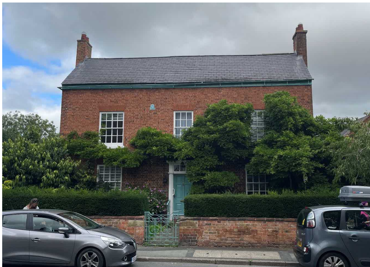
Figure 12: Principal elevation of 73 High Street
